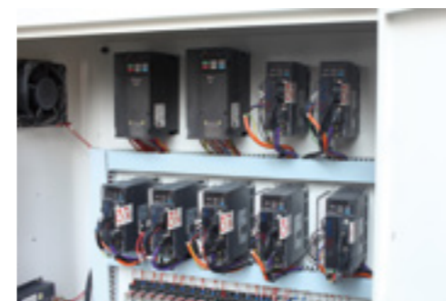
Taiwan Delta drive system, imported electrical components
